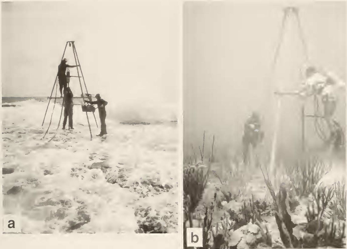
Figure 6. Working with hydraulic-operated coring equipment: (a) Above water drilling the Holadés Ridge, Panamá. 1993. (b) At a depth of 15 meters, coring a relict reef off the southeast coast of St. Croix. 1976.
